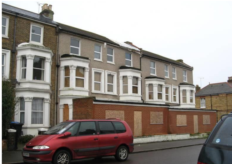
Inappropriate 'build-outs' in Sweyn Road
